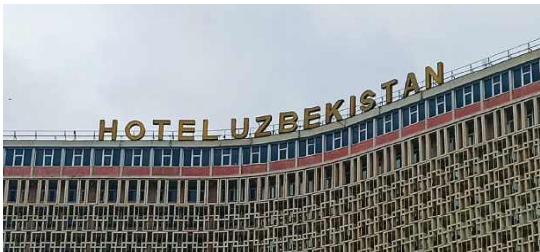
Taszkent, Hotel Uzbekistan
