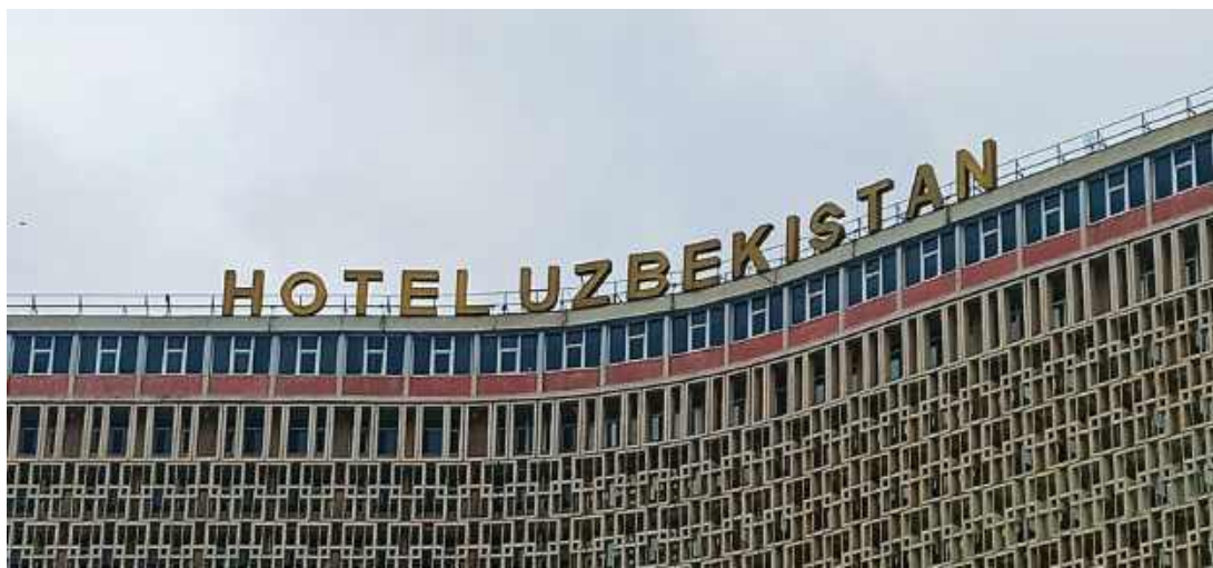
Taszkent, Hotel Uzbekistan
