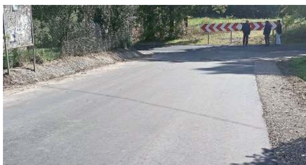
Nowa droga w Pohulance
