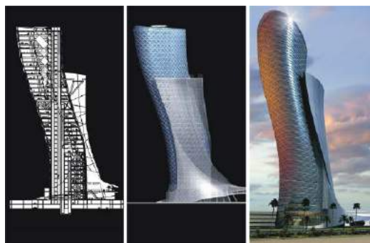
1. Capital Gate Tower
