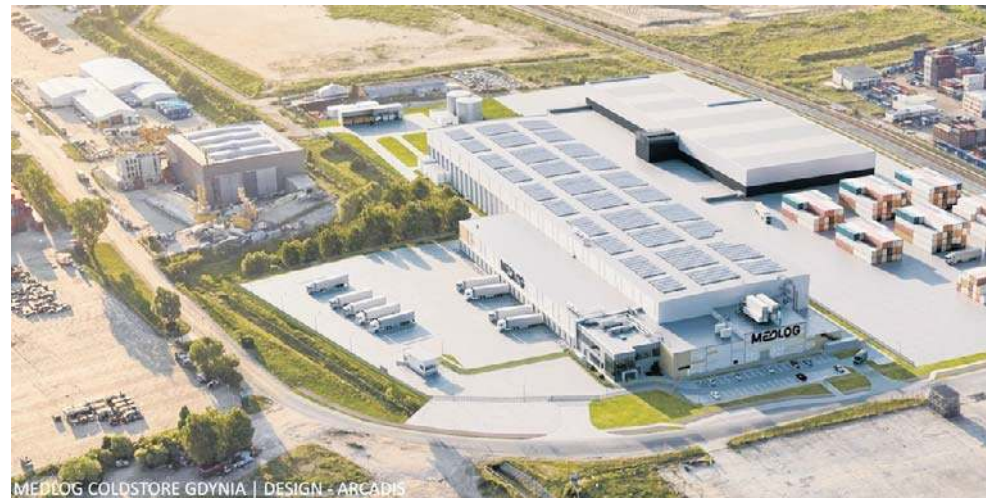
MEDLOG COLDSTORE GDYNIA | DESIGN - ARCADIS
