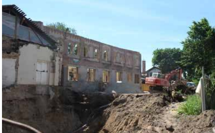
Remont TCDK - lato 2014
